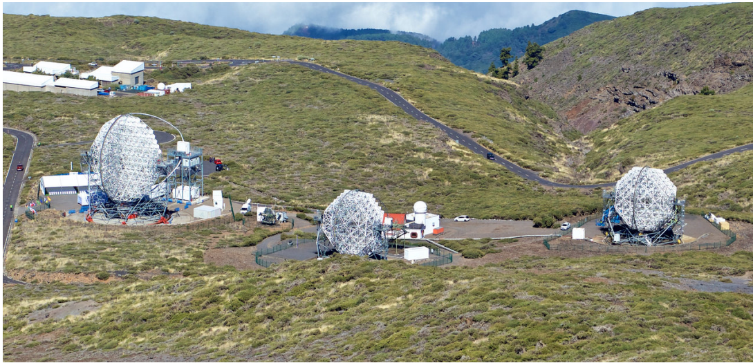
Figure 1: Visible in the photograph, from left to right, the first Large Size Telescope of CTA LST-1 of 24 m mirror-diameter, FACT (4 m) and the MAGIC telescopes (12 m) at Los Roches de Muchachos, La Palma. The LST-1 was inaugurated on Oct. 2018.
