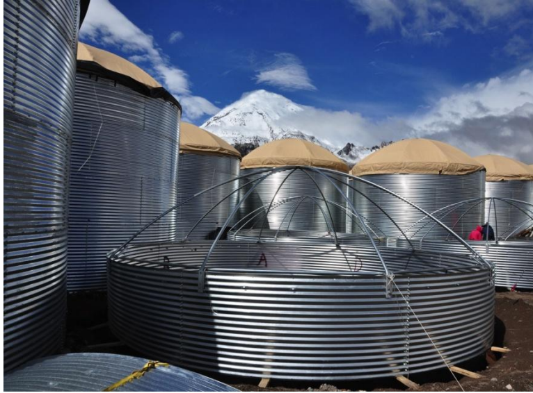
Commercial steel tanks constructed at the site.
