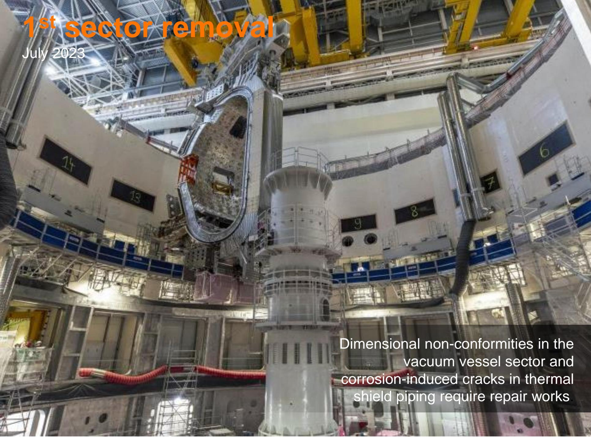
Dimensional non-conformities in the vacuum vessel sector and corrosion-induced cracks in thermal shield piping require repair works
