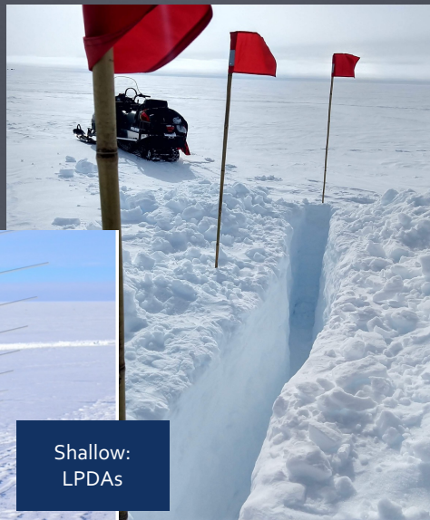
Shallow antennas deployed in trenches
