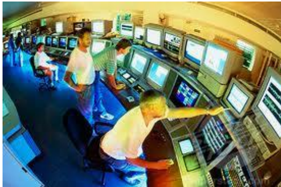
DESY's control room (Germany)
