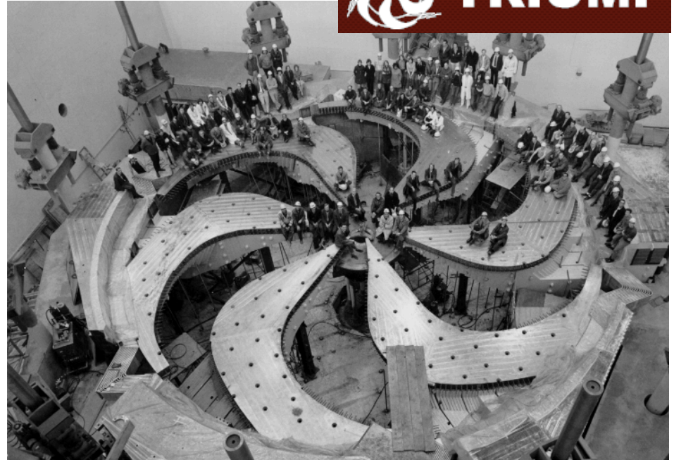
Cyclotron magnet and staff, 1972
