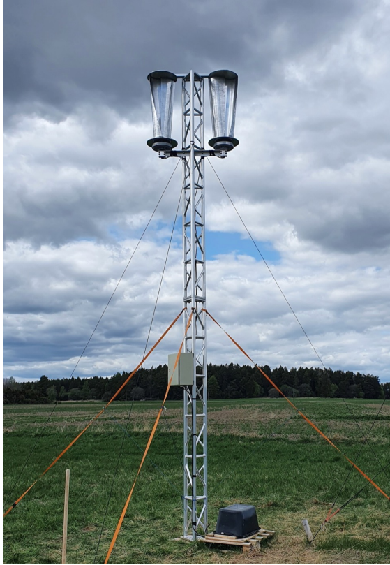
Wind turbine developed at Uppsala - 3 stations sent to Greenland for RNO-G
