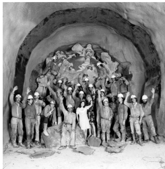
SPS tunnel ready 1974
