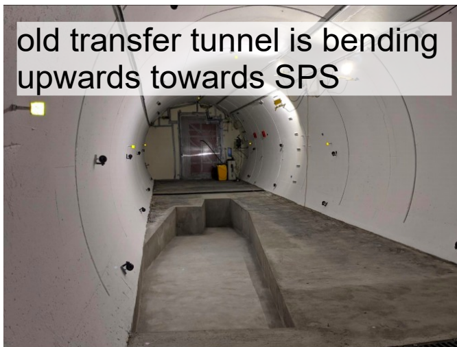
04/2020 modification of the tunnel floor
