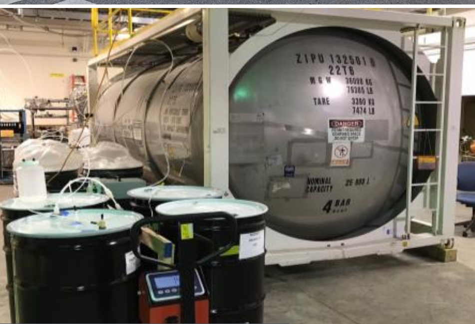
Filling from Mixing Tank
