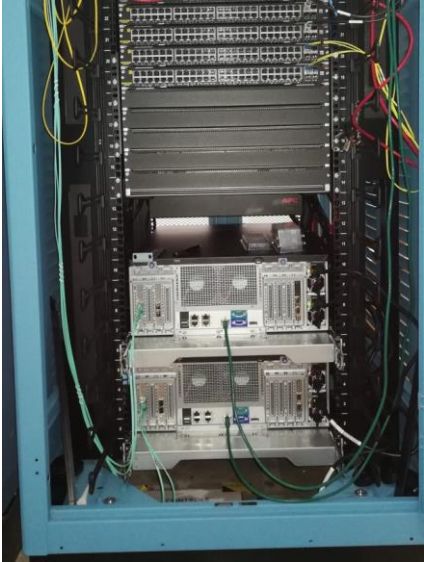
Example of DAQ Linux Servers installed
