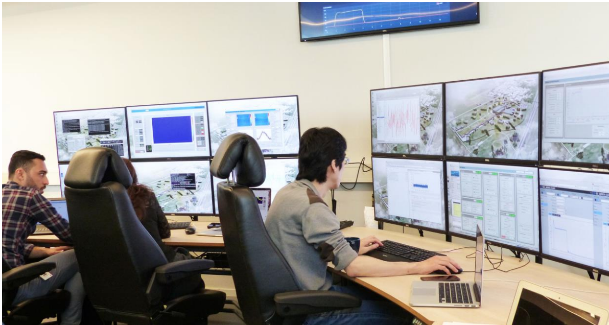
Temporary Control Room (Final control room will be in target building, not ready yet)
