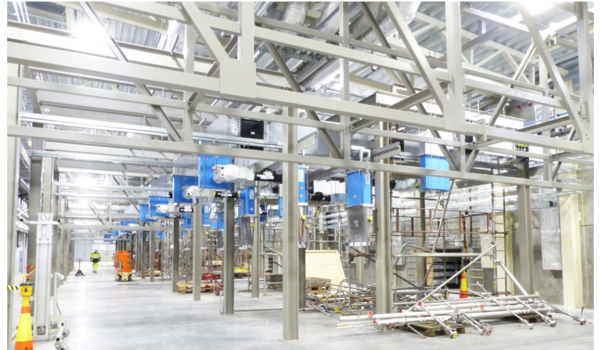
RF Waveguides and loads are being installed
