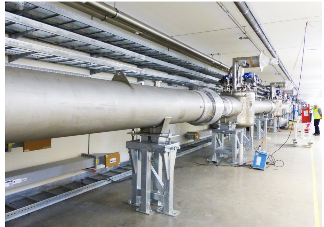
Cryo distribution lines being installed. The tunnel starts to feel tight...
