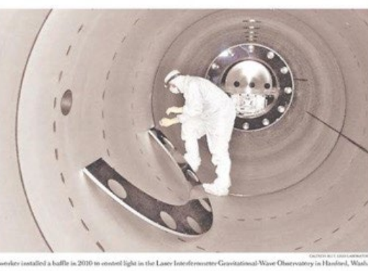
A worker installed a baffle in 2010 to control light in the Laser Interferometer Gravitational-Wave Observatory in Hanford, Wash.
