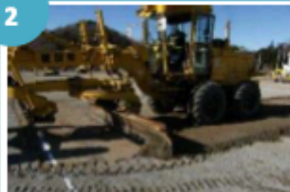
●Scraping off of topsoil of school yards (Provided by JAEA)
