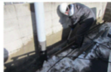
●Removal of sludge from ditches (Provided by Fukushima City)
