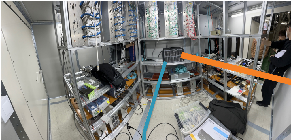
Faraday cage under construction
