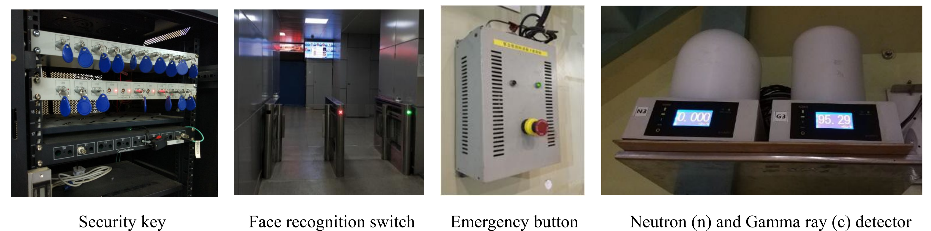
All the statuses are integrated in the central safety and interlock system
