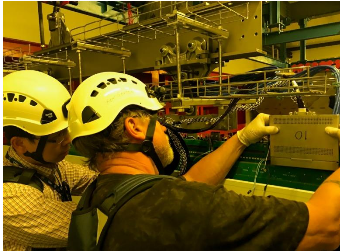
Install CE boxes on the top of APA
