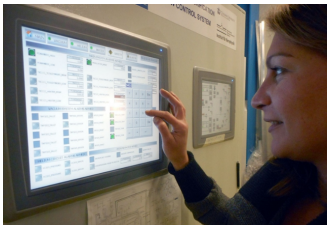
Operator at local touch-panel (Beijer Exter T150) setting alarm thresholds
