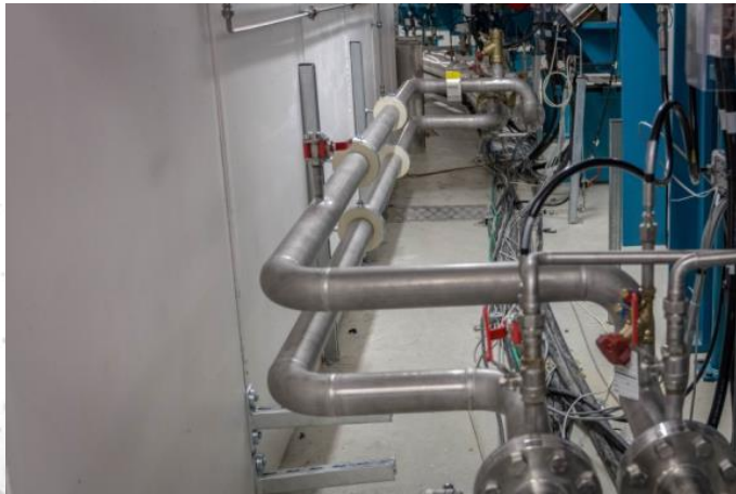
New 30°C cooling circuit
