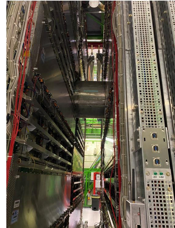
Beam pipe shielding crossing the MID
