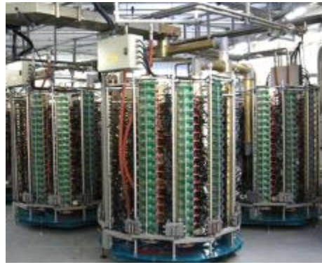
SOLEIL Storage Ring : 4x45 kW, SSPA (operation from 2006)
