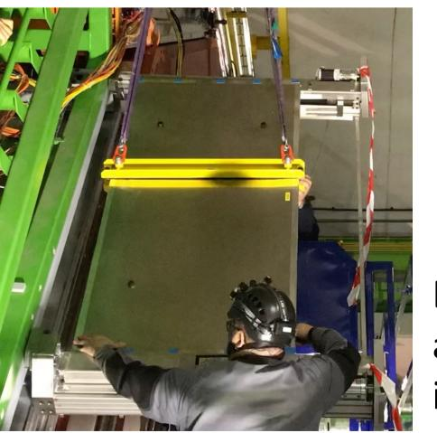
Lead + borated polyethilene shielding cassettes installed in all top sectors
