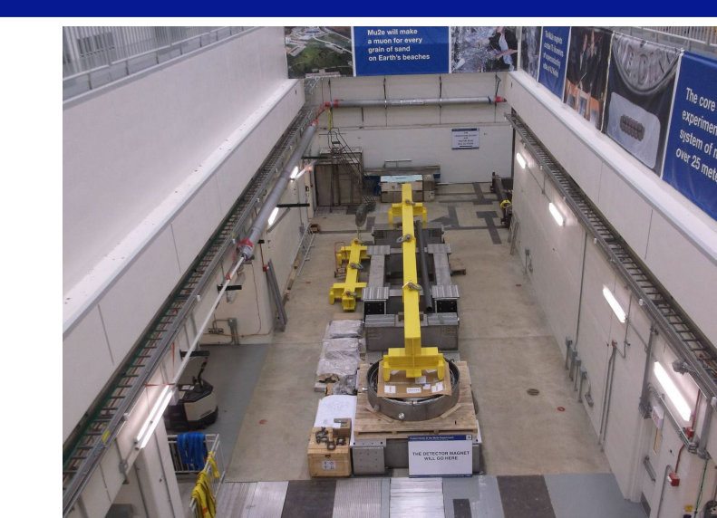
Mu2e experimental site in construction @ Fermilab
