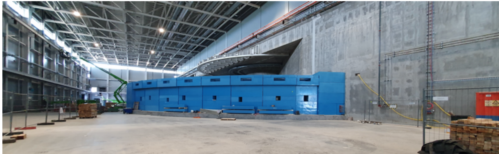
Neutron Bunker construction of North and west sector D03
