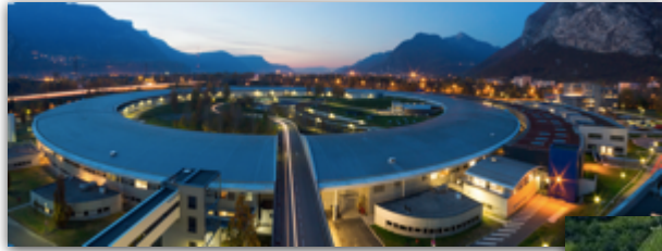
MBA upgrades SR
