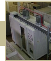
Main magnet chokes and DC PSU
