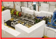
Collector straight replacement
