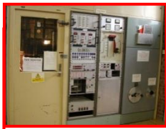
Linac modulator 3 and 4 refurbishment
