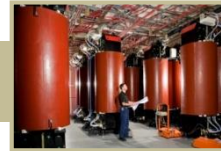
Main magnet chokes and DC PSU
