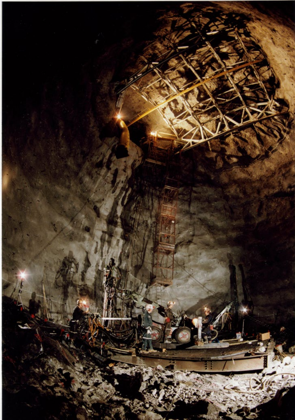
Start of construction of PMT support
