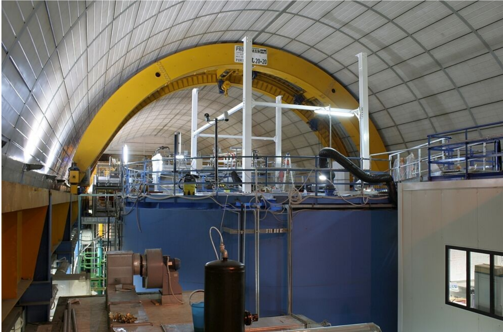
20-ton overhead crane, 1 kton water Cherenkov veto tank (before DS-50 support structures installed)
