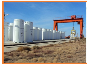
Spent Fuel monitoring
