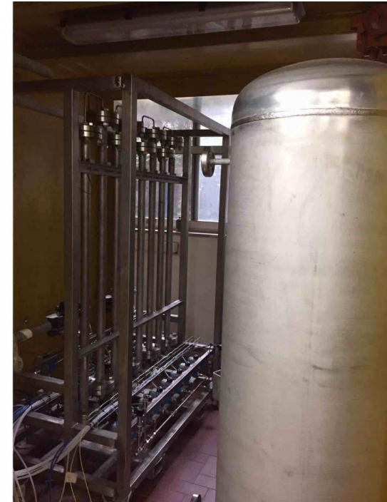
Development of Urania underground argon extraction facility
