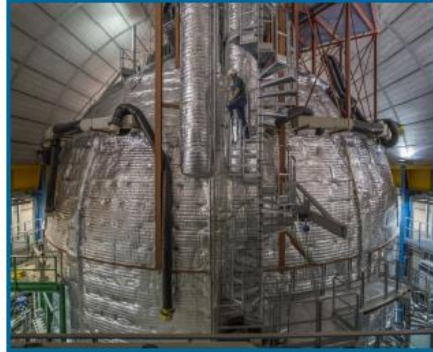
After thermal insulation
