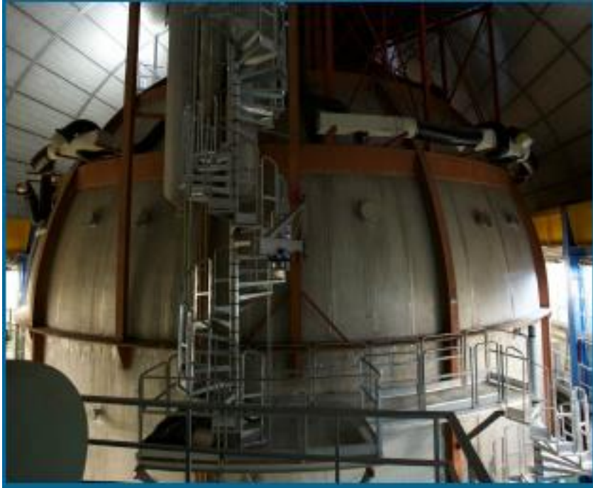
Before thermal insulation
