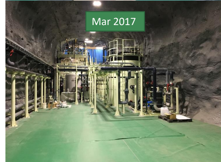
New water system 8 m x 7 m x 50 m
