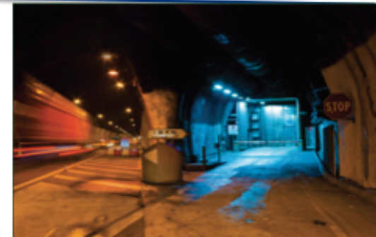
Entrance to underground labs
