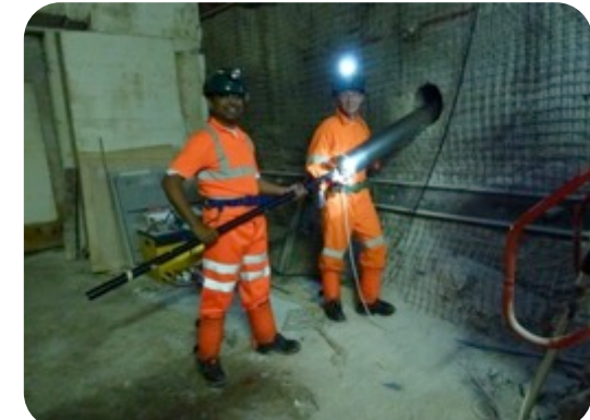
Bore hole detector installation
