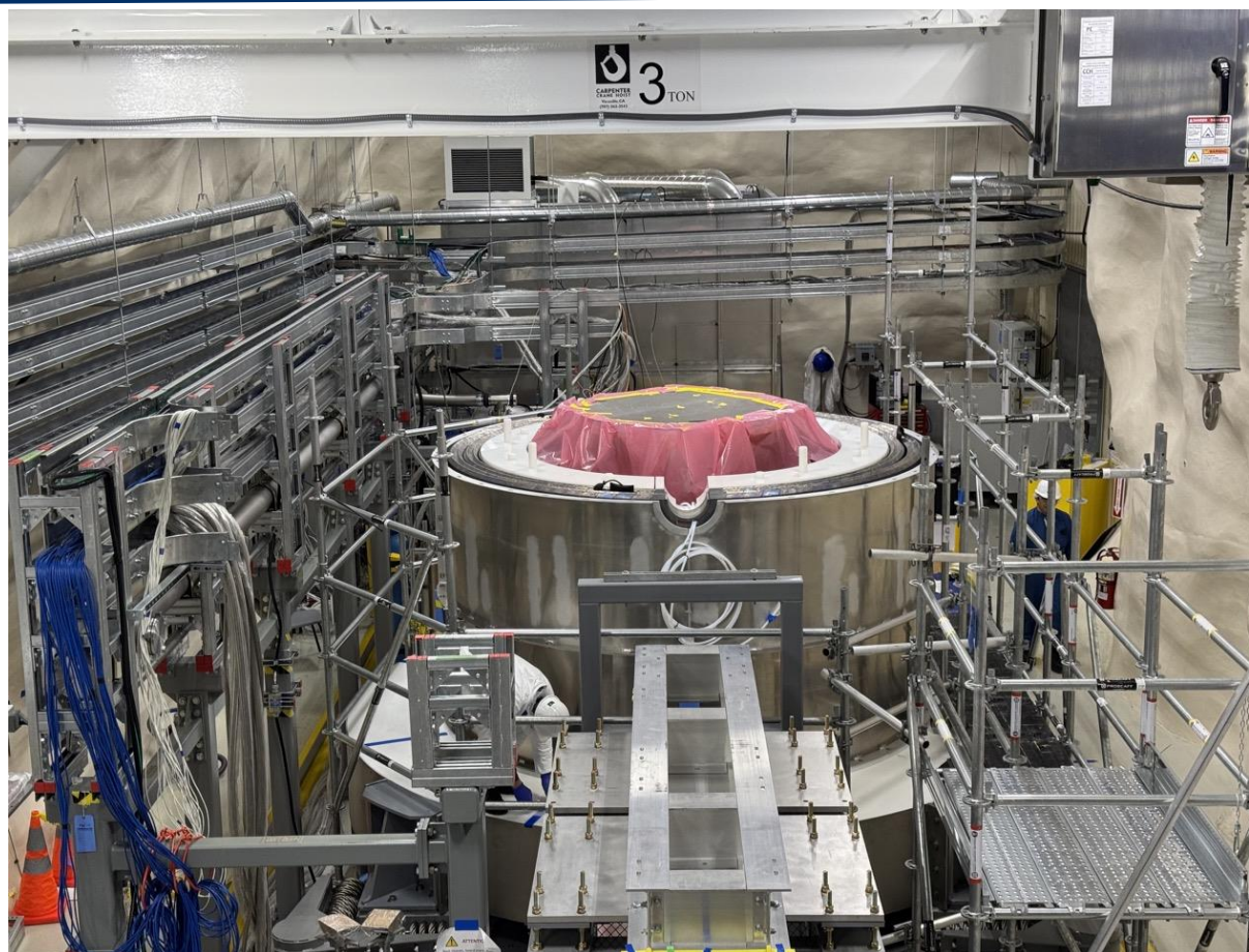
March 2025 Shield wall 2/3 complete
