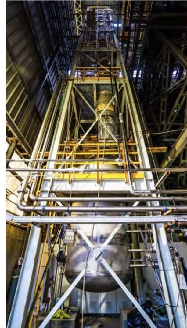
Column before deployment
