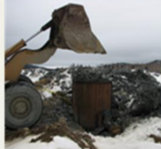
Using a scooptram to knockdown the frozen column
