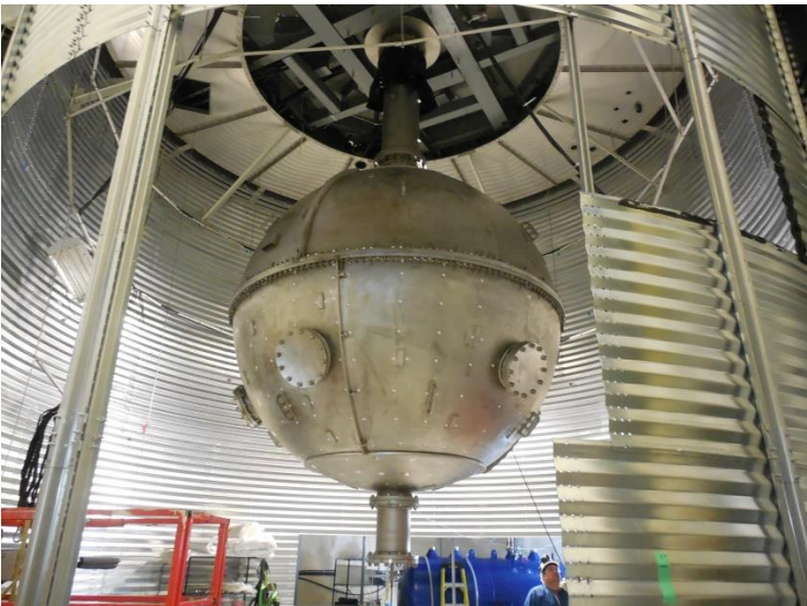
Steel Shell in shield tank
