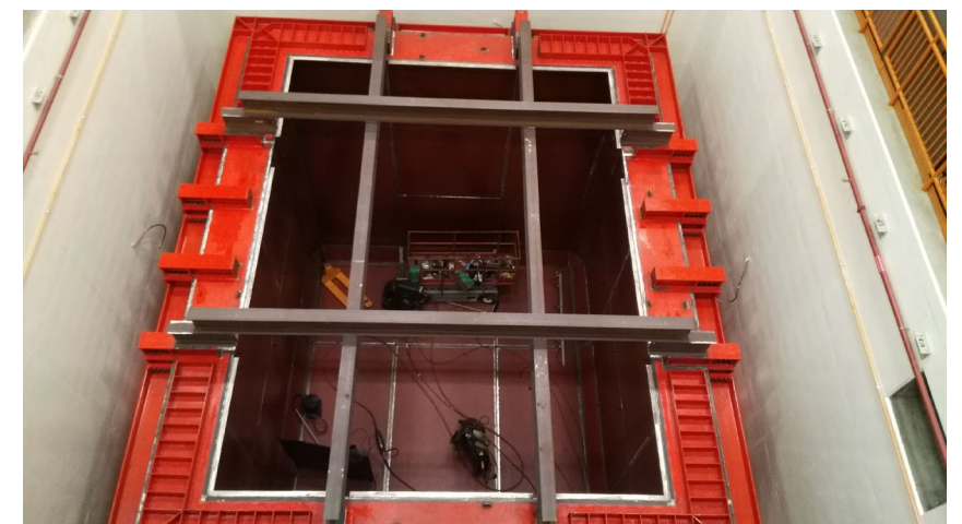
Outer frame for cryostat
