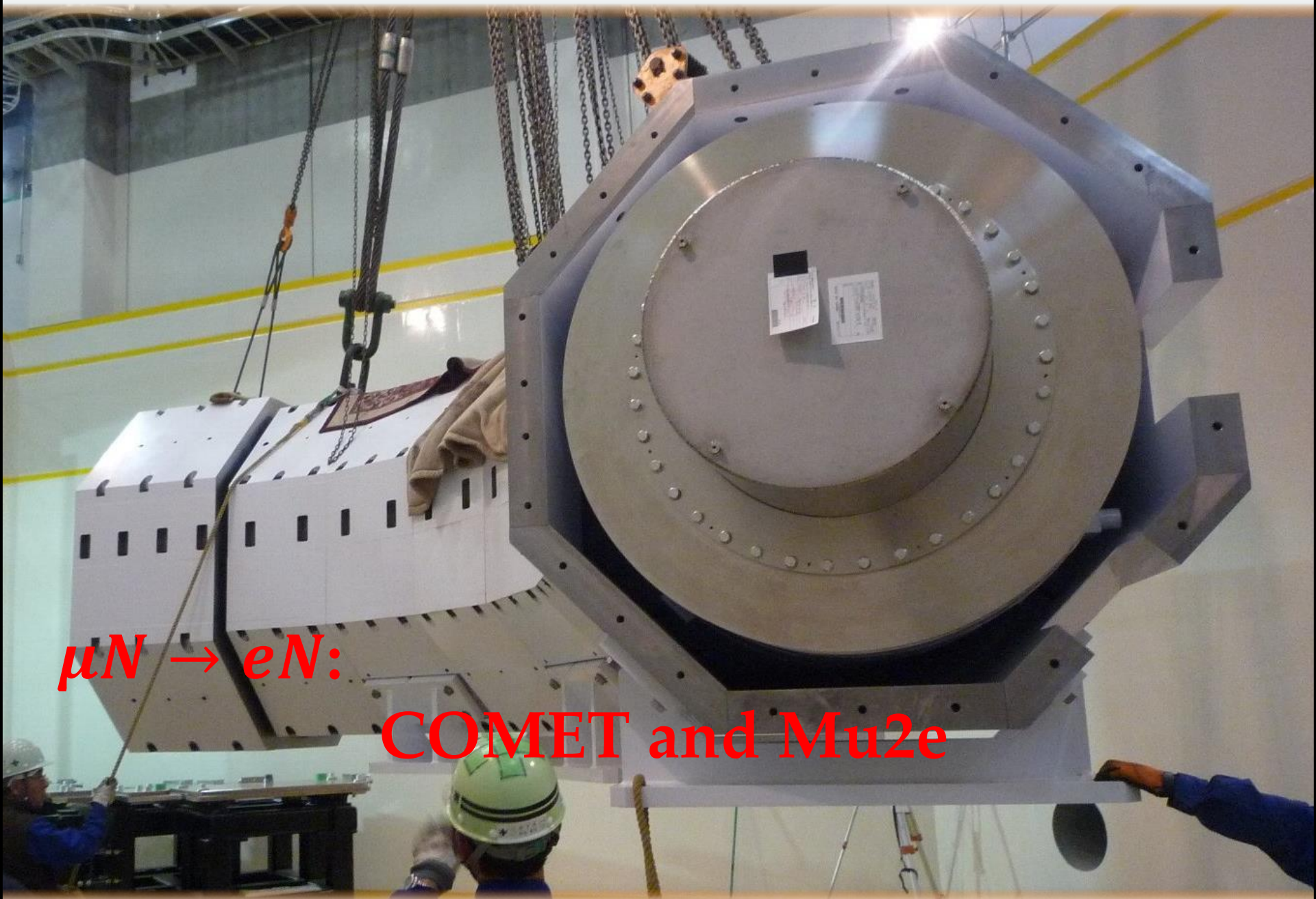
Lowering the 1 st COMET transport solenoid into place
