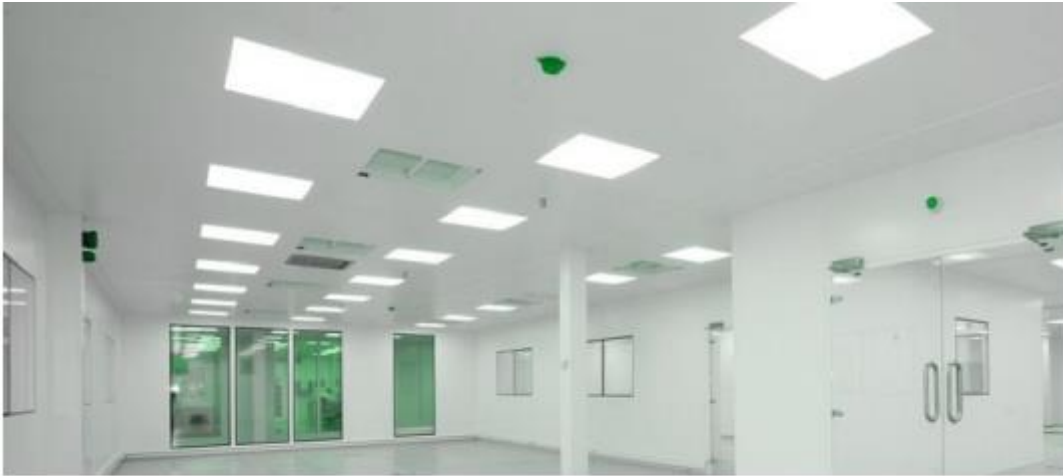
BEST PRACTICE - FLUSH LIGHT FITTINGS AND INTEGRATED SERVICES
