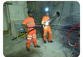
Bore hole detector installation
