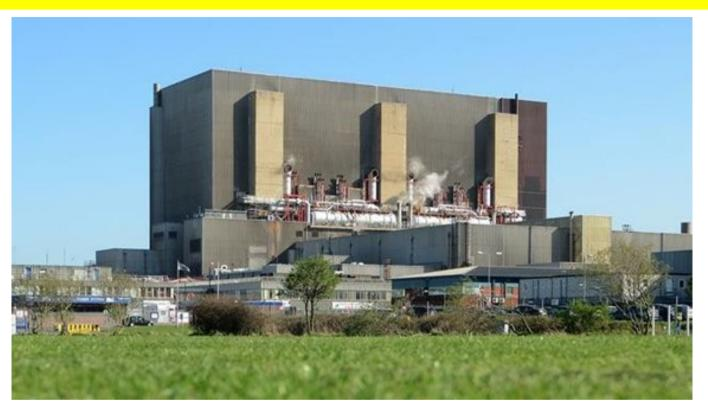
Dual-core reactor complex Advanced gas-cooled reactors (AGR) 1550 MW<sub>th</sub> per reactor core
