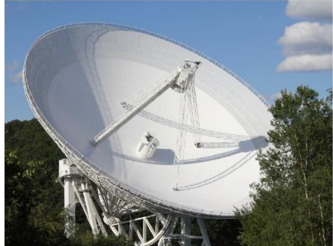
The Effelsberg d=100\text{m} , f=30\text{m} radio telescope in Germany
