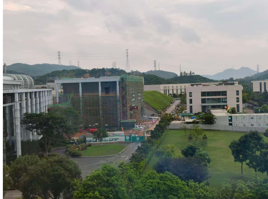
Construction of experimental hall
