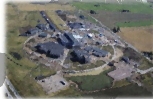
ESS (under construction)
