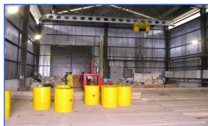
Radioactive waste storage facilities (5A)
