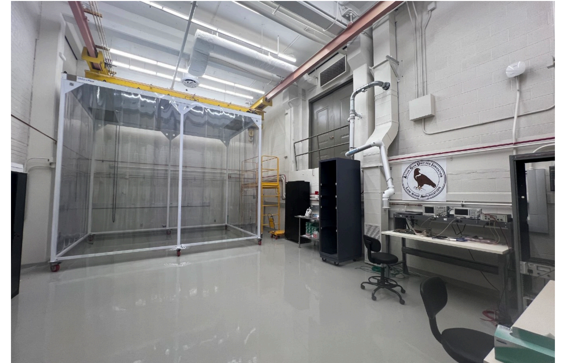
Lab space with ISO 7 cleanroom and crane
