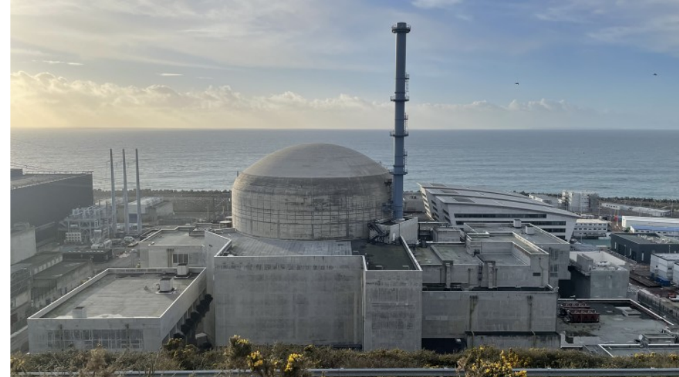
EPR, Flamanville, France (Gen III+, 1300MWe)
