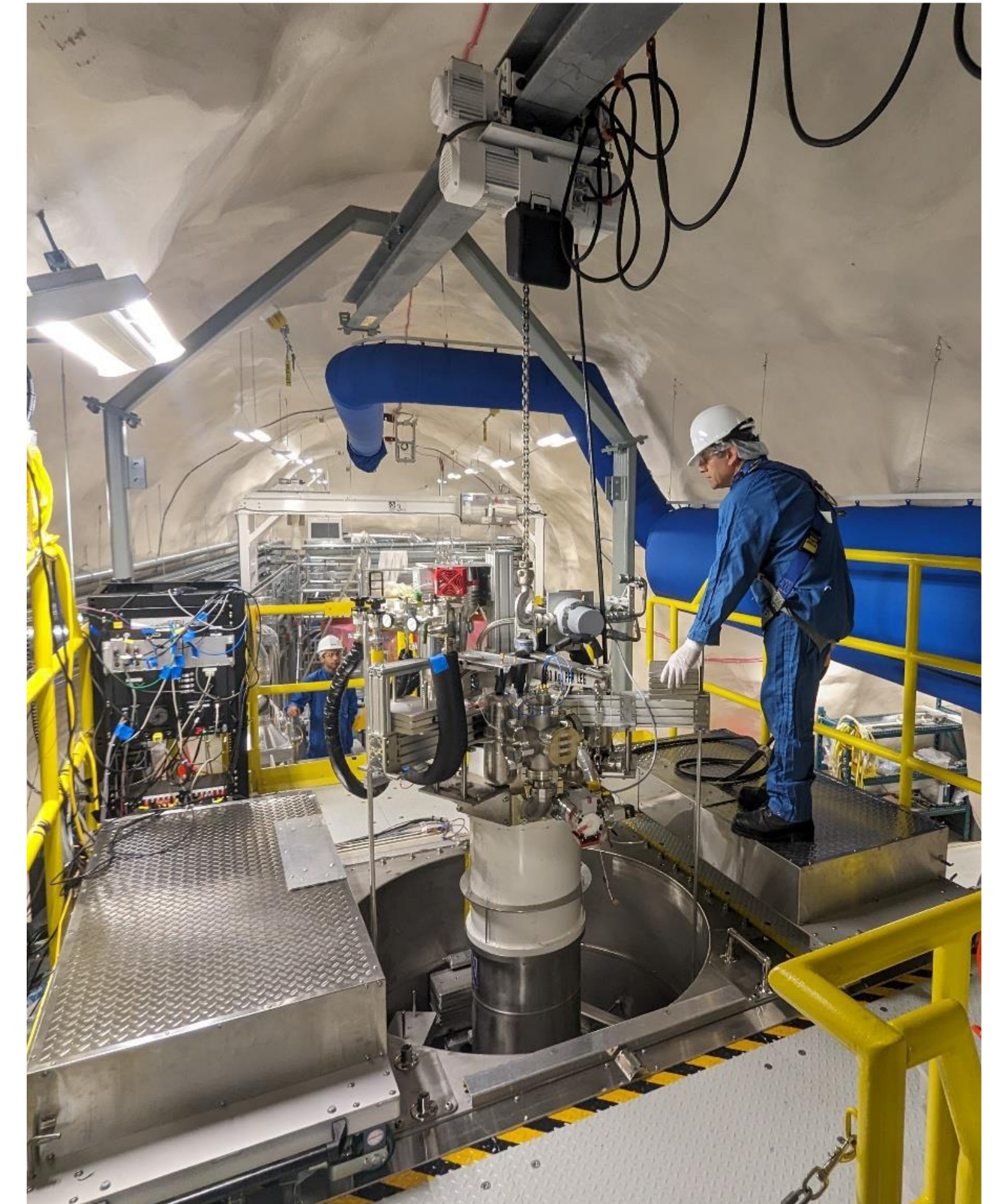
Lowering of DR into drywell
