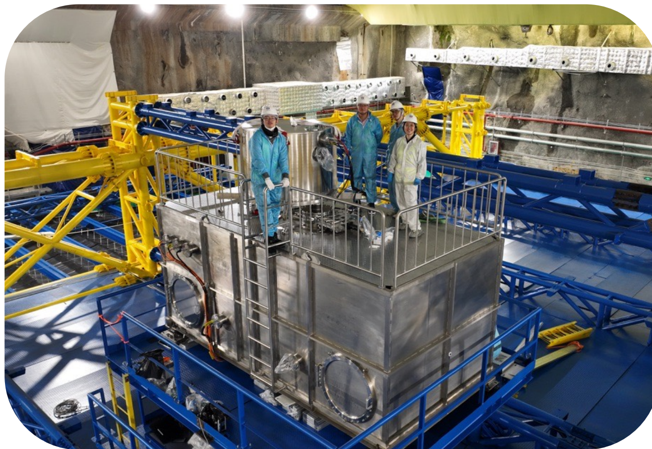
Calibration house on top of the detector
